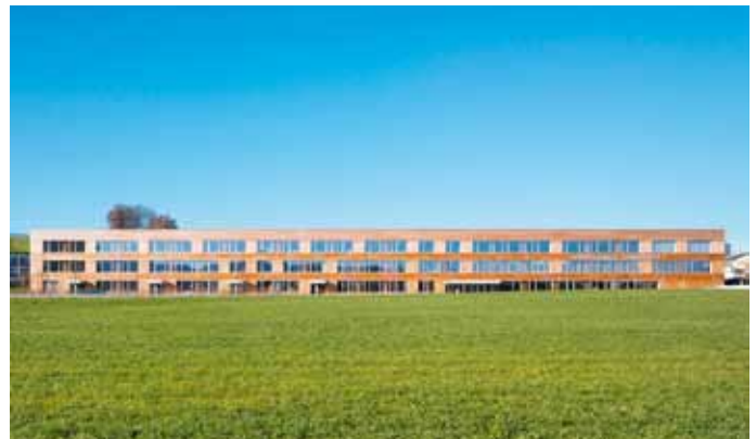
Langgestreckter Schulneubau in Hybridbauweise. Stretched new school building in hybrid construction.
